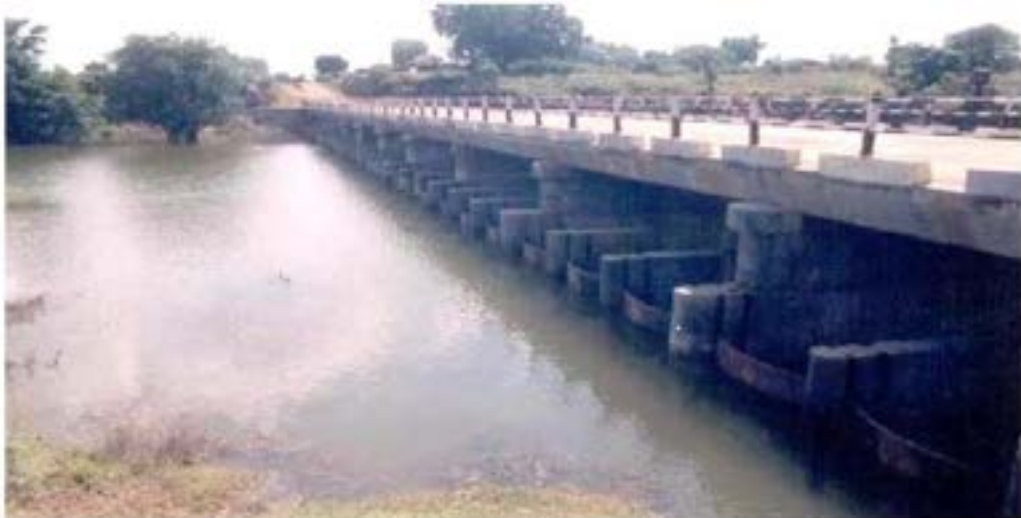
Figure 1. Bandhara/Barrage Structure constructed on Addan River, Distt. Yawatmal, Maharashtra (MoRTH,2017)
