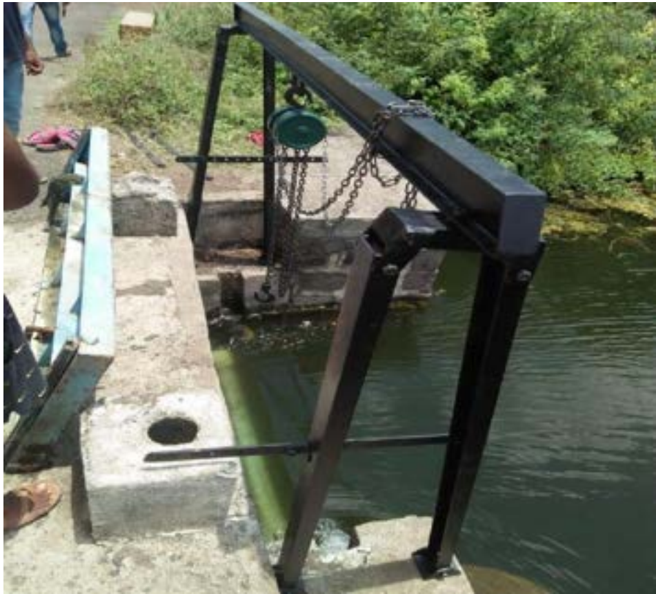
Figure 2 Proposed and installed mechanism
