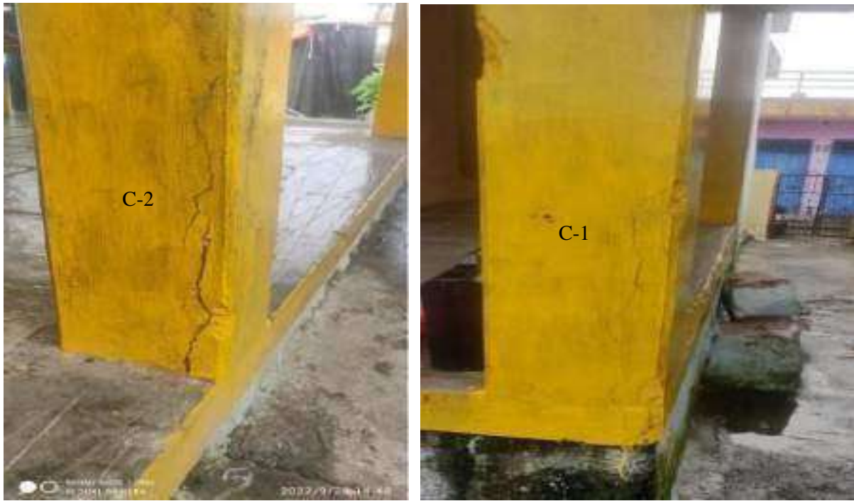
Fig 5: Column with major cracks
