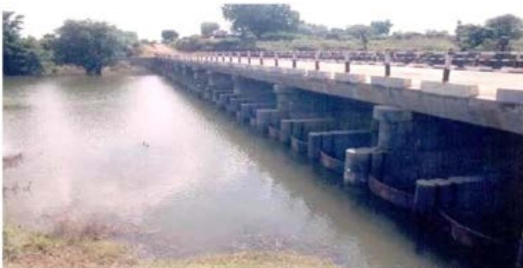
Fig.2 –Bandhara/Barrage Structure constructed on Addan River, Distt. Yawatmal, Maharashtra (MoRTH, 2017)
